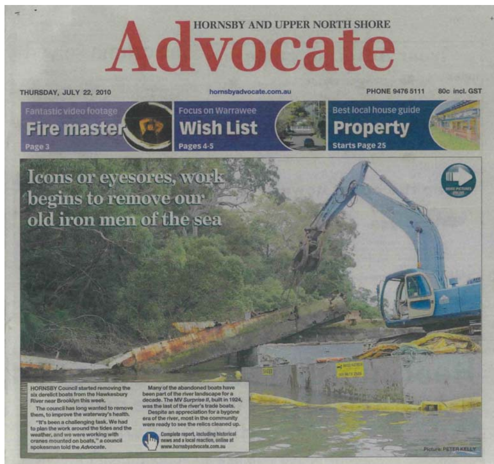
Figure 1: High profile projects undertaken include the removal of derelict boats from Sandbrook Inlet
