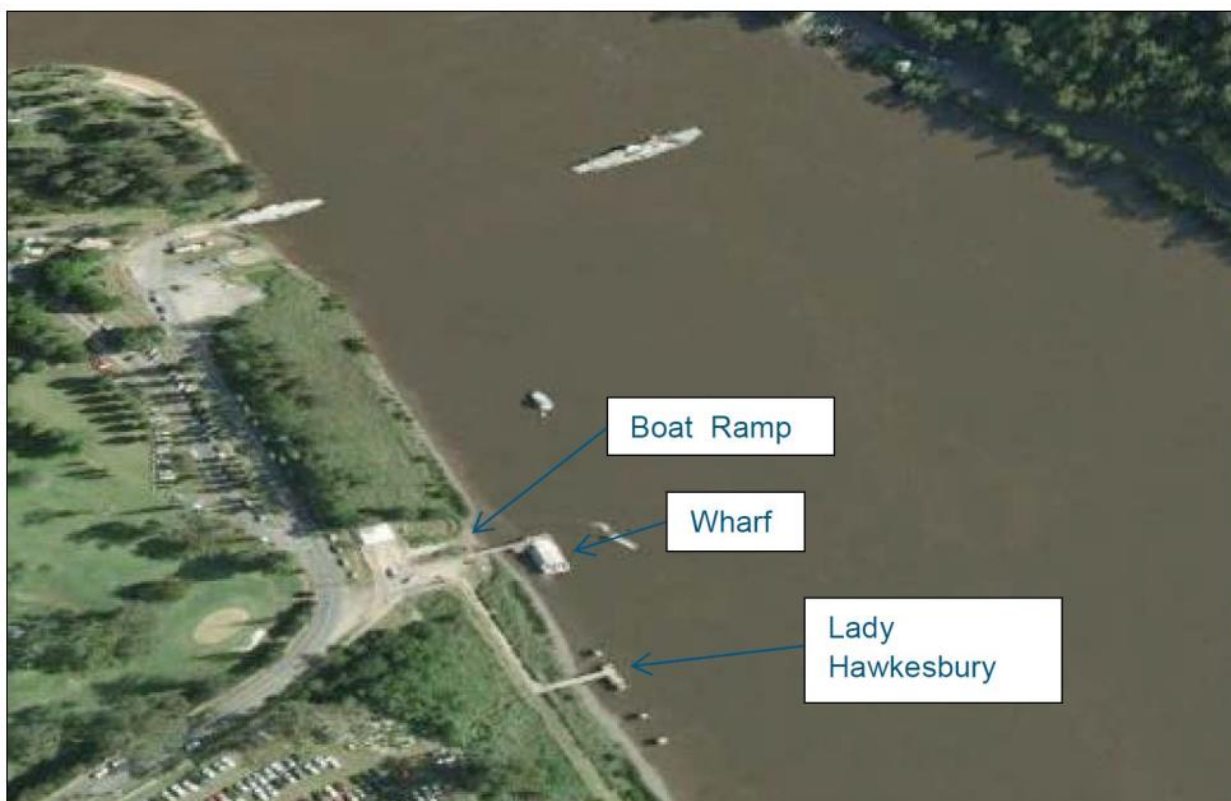
Figure 1: Location of existing boat ramp
