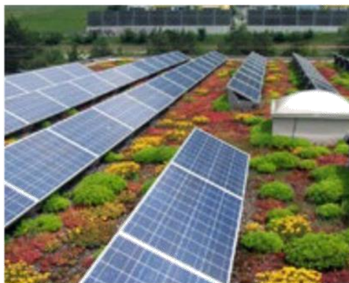
Solar panels have improved efficiency when used in combination with green roofs (Source: OEH publication – Urban Green Cover in NSW)
