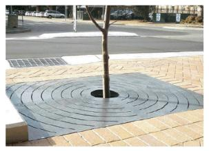
Image C.13: Installed bioretention tree grate in brick paving Coronation Street, Hornsby
