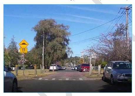
Figure 2-19: Balmoral Street raised platform and kerb widening
