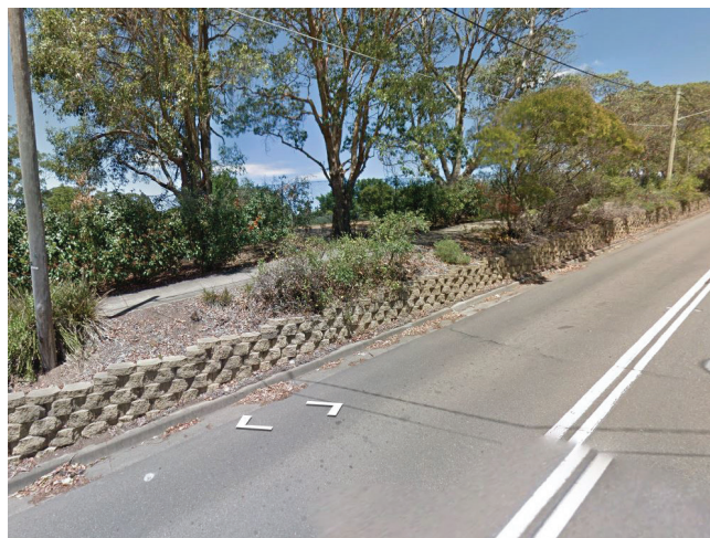
Figure 23: Retaining wall on verge
