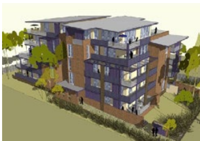
Figure 3.4(e): Building Height. (l) Height controls are based on a typical residential floor to floor height of 3 metres, with a 1.5 metre allowance for roof articulation and a 1 metre basement projection.
