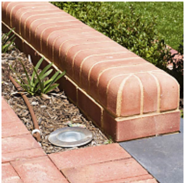
road reserve garden edges LOW BRICK WALLS with bullnosed header. Brick colour + details to match existing walls on Beecroft Rd
