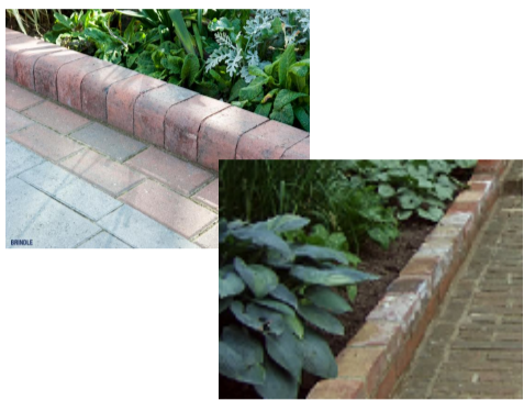
sunken court garden edges LOW NARROW BRICK EDGE 110mm wide with optional bullnosed capping edging to sandstone paving (See Detail)
