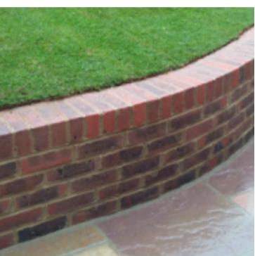
garden walls - driveway entry LOW BRICK WALLS Brick retaining walls finished to design levels. Material to be selected brick to match existing red brick on site, capped with 230mm header course.
