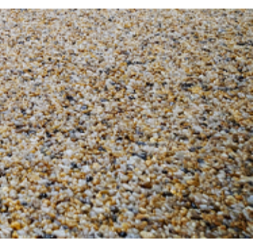
porous paving T.P.Z. CAFE COURTYARD Porous paving similar to StoneSet to be installed under canopy T54 Ulmus parvifolia in accordance with Arborist Report
