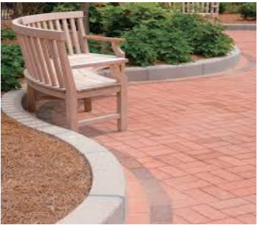
cafe courtyard garden edges CURVED CONCRETE EDGING Low edging (150mm high) tinted with light grey-brown pigment to match selected stone + architectural trims.
