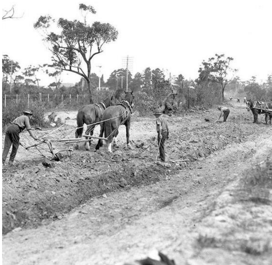
Construction of the Pacific Highway near Berowra, c1925. (Source: Hornsby Shire Recollects)
