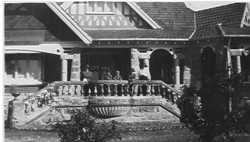
The main entrance to Mount Wilga, built by Marcus Clark, 1923. (Source: Hornsby Shire Recollects)
