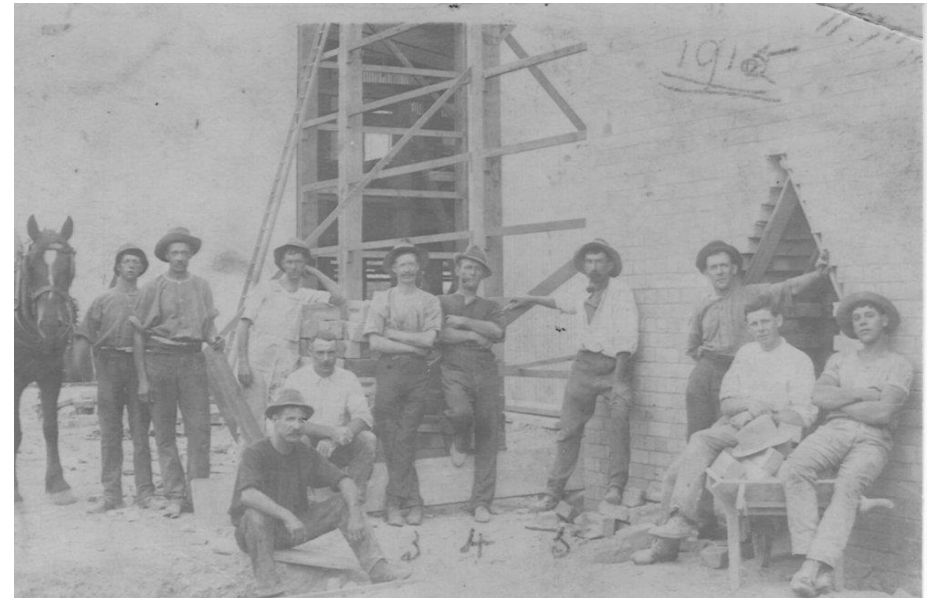
Workers constructing one of the large chimney stacks at the Hornsby Tile, Pottery and Brickworks, 1915. (Source: Somerville Collection, Hornsby Shire Recollects)
