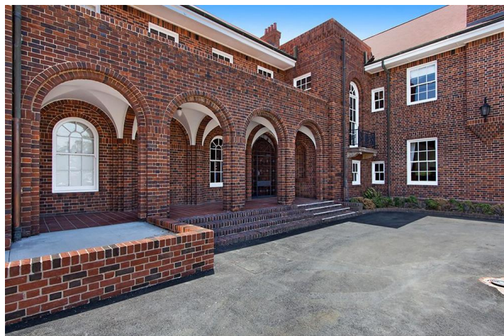
Castle Hill Mowll Memorial Village (Lober House). (Source: Tower Projects)
