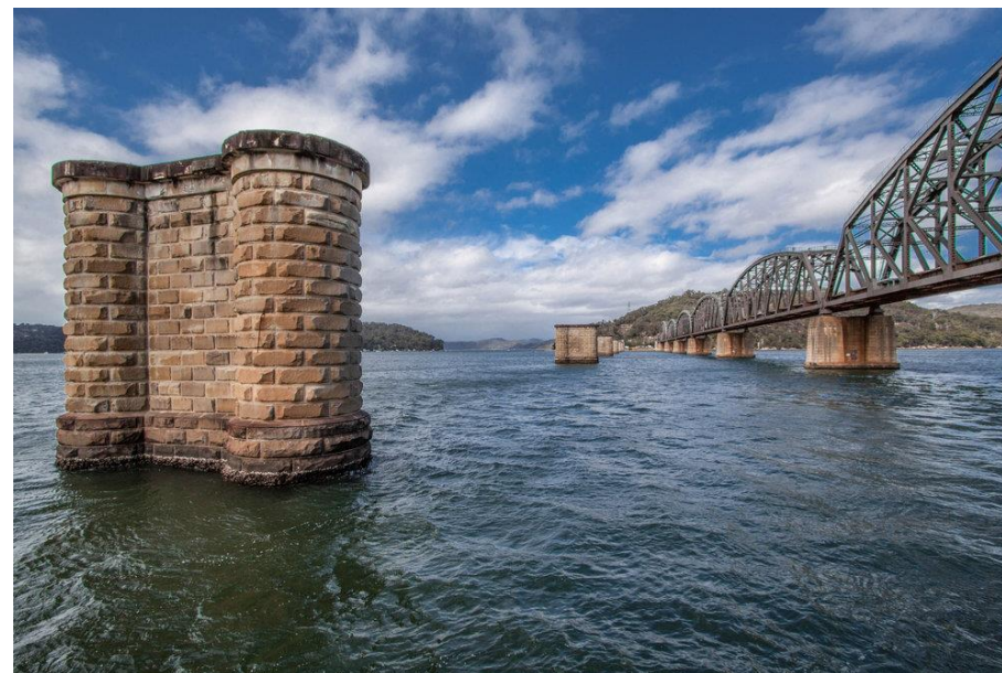
Second Hawkesbury River Railway Bridge alongside the pylons from the first railway bridge, 2012. Photograph by Robert Green. (Source: Hornsby Shire Recollects)
