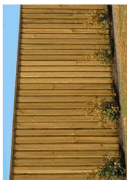
1.8m tall timber fencing to side and rear boundaries typically lapped and capped as recommended by acoustic report.
