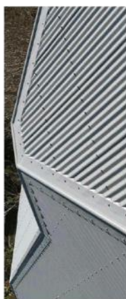
Roof cladding: corrugated metal roof sheeting in colorbond colour: "Basalt".
