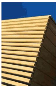
Timber-lock aluminium vertical battens to front elevation.
