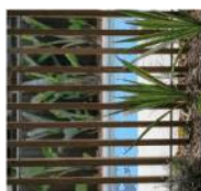
Front yard external play area fencing: posts with clear polycarbonate infill panels. On driveway side, 60% open vertical timber battens to be added to external face.
