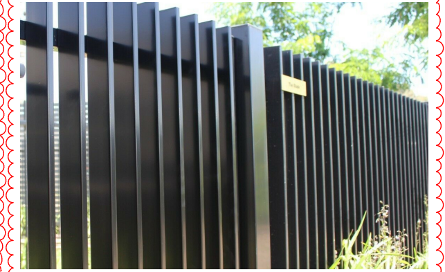
Charcoal coloured (Colorbond Monument) aluminium vertical battens to front elevation.
