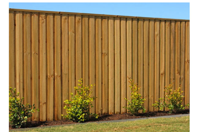
1.8m tall timber fencing to side and rear boundaries typically. Lapped and capped as recommended by acoustic report.
