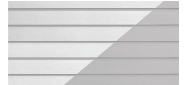
Painted fibre-cement weatherboard cladding typically to upper level external walls.
