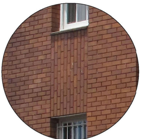
VERTICAL BRICK UNDER WINDOW DETAILING
