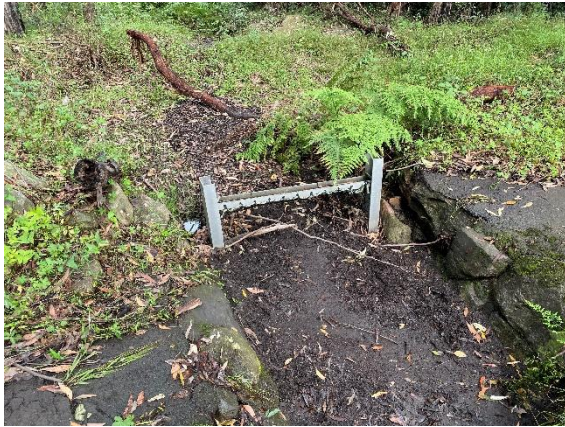
Figure 11: Full gross pollutant trap below Britannia Street
