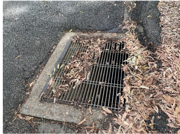
Figure 12: Leaf litter entering stormwater drain on Malton Road
