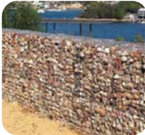
Low Welded Mesh Gabion Wall
