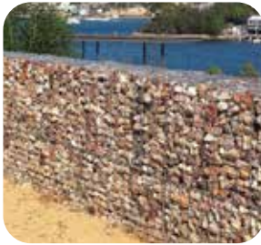
Low Welded Mesh Gabion Wall
