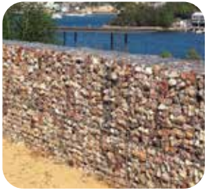
Low Welded Mesh Gabion Wall
