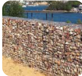
Low Welded Mesh Gabion Wall
