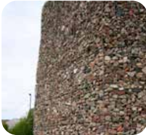
Sandstone Welded Mesh Gabion Wall
