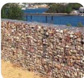
Low Welded Mesh Gabion Wall
