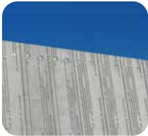
Off-form Concrete Wall
