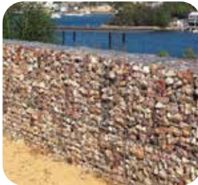
Low Welded Mesh Gabion Wall
