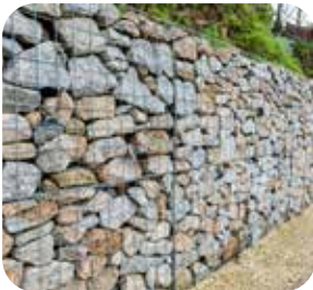
Breccia Welded Mesh Gabion Wall
