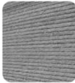
Raked Concrete Footpath
