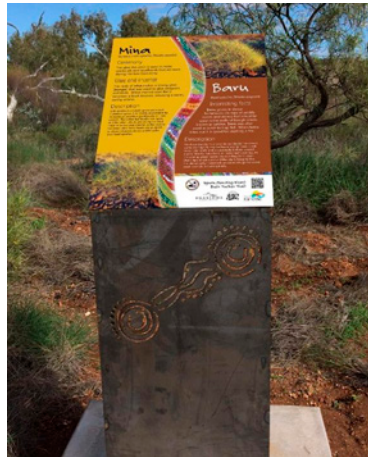
c) use of Corten (rusted steel) for supports
