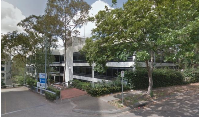
Figure 7: Commercial office building on the site, viewed from City View Road (Source: Google).
