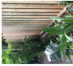
Lapped and capped timber side & rear boundary fencing, 1.8m tall.
