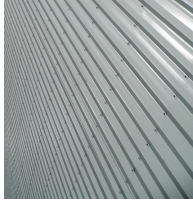
Metal Roof sheeting
