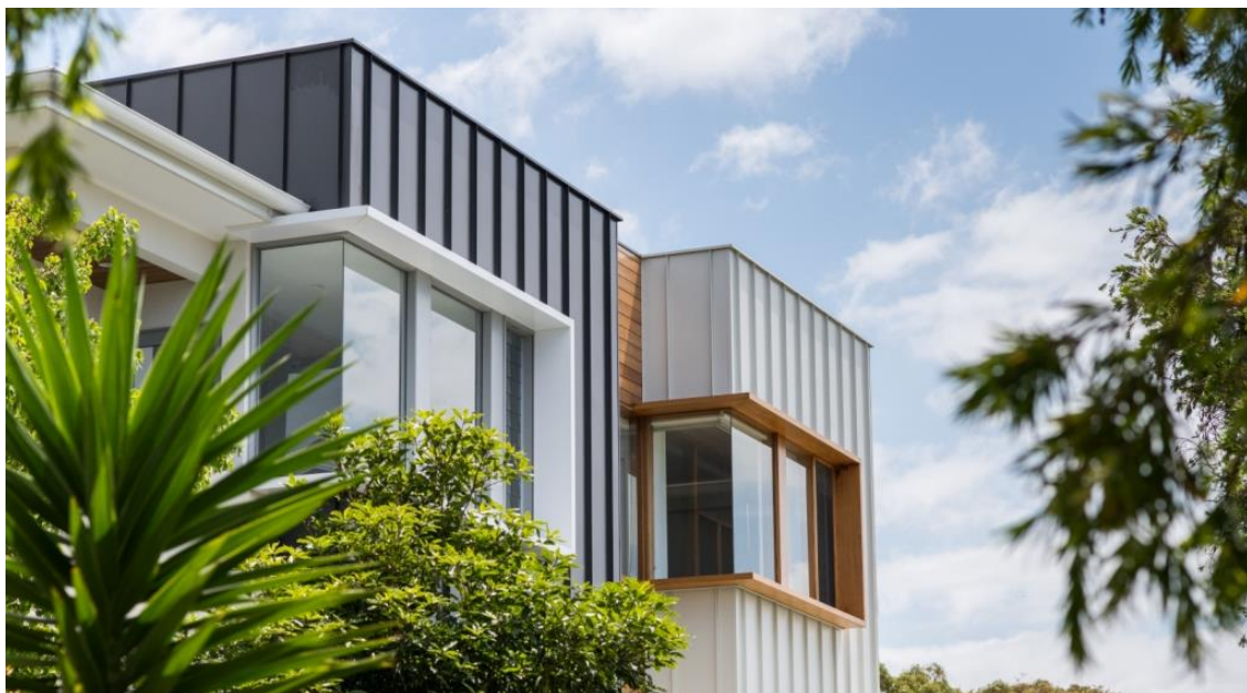
Figure 2: Dual occupancy Cronulla – Jamisa Architects
