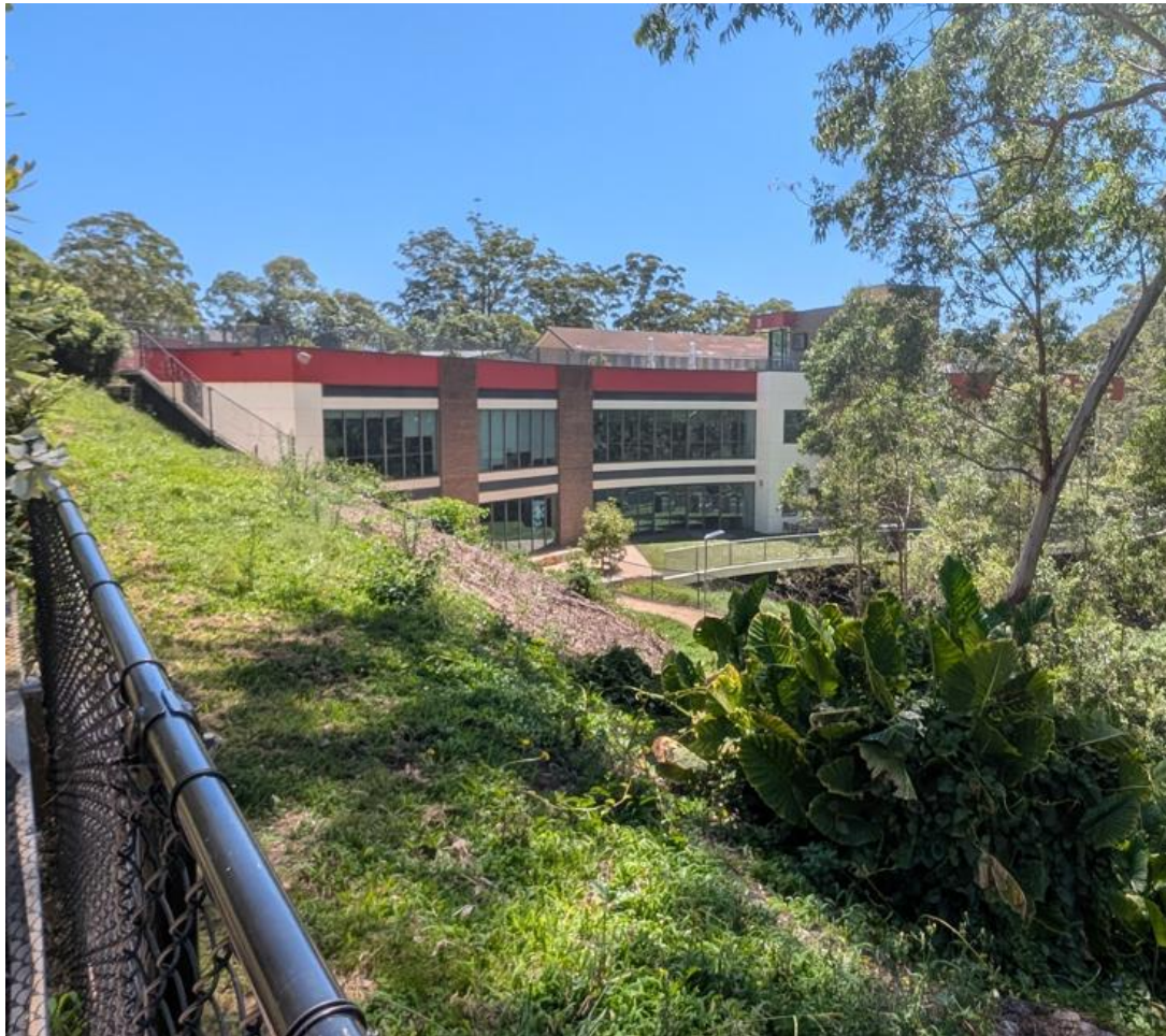
Figure 5: Site photo of existing Hildegard Centre looking towards the south elevation (Source: HSC)
