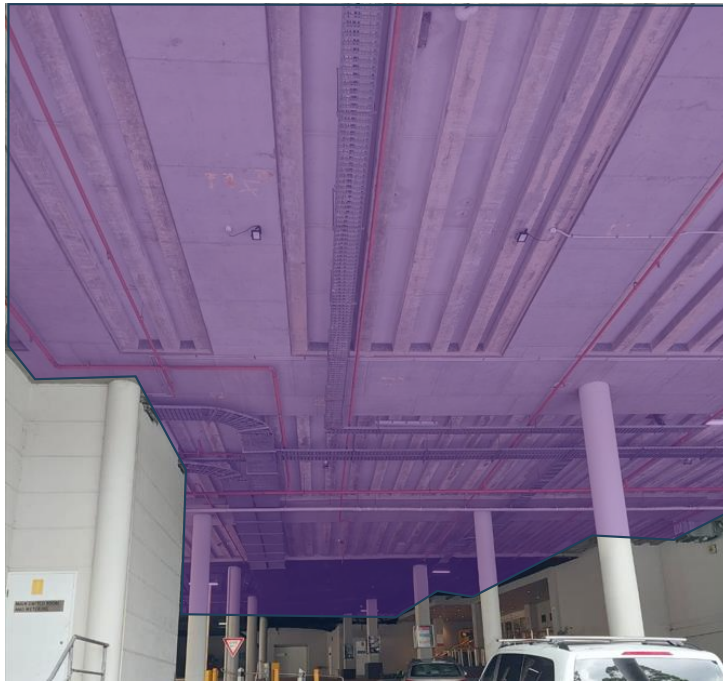
Figure 6-2 Acoustic absorption (NRC 0.7) to be applied to Carpark ceiling
