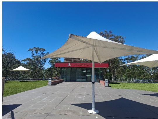
Picture 4 Existing rooftop open space next to Hildegard Building
