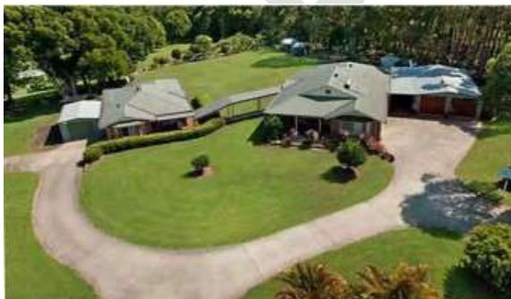
Figure 2.2-b: Covered walkways are not acceptable means of attaching the two dwellings (E)
