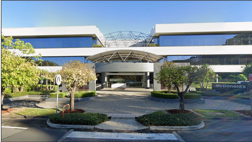
Figure 1: Eastern parcel of land at 21-31 Central Avenue as viewed from Central Avenue facing east (Google Maps 2025)
