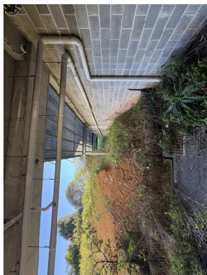
Image 03 - View from basement undercroft area looking North along retaining wall and steel walkway above
