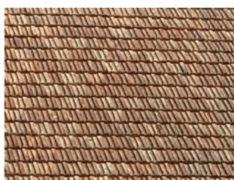
Terracotta roof tiles. Salvage and reuse where possible
