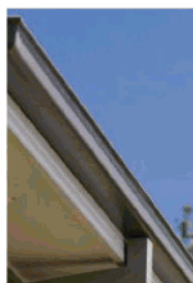
Colorbond, gutter, fascia and downpipes. Jasper colour to match existing
