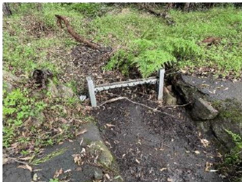
Figure 11: Full gross pollutant trap below Britannia Street
