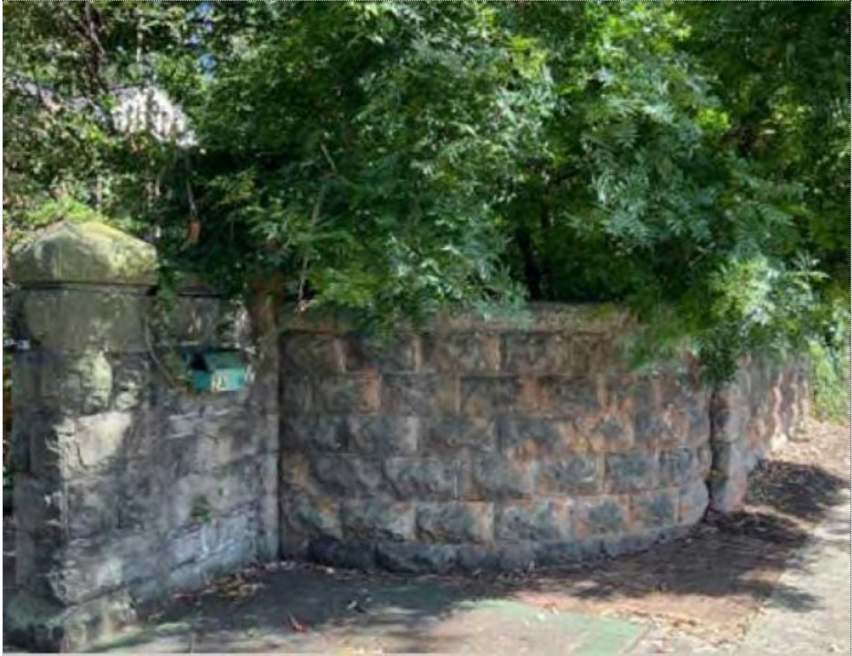
Sandstone block fence and entrance at 2A Beecroft Road.
