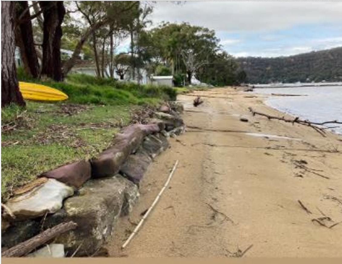
Section of sandstone rubble lining the easement.
