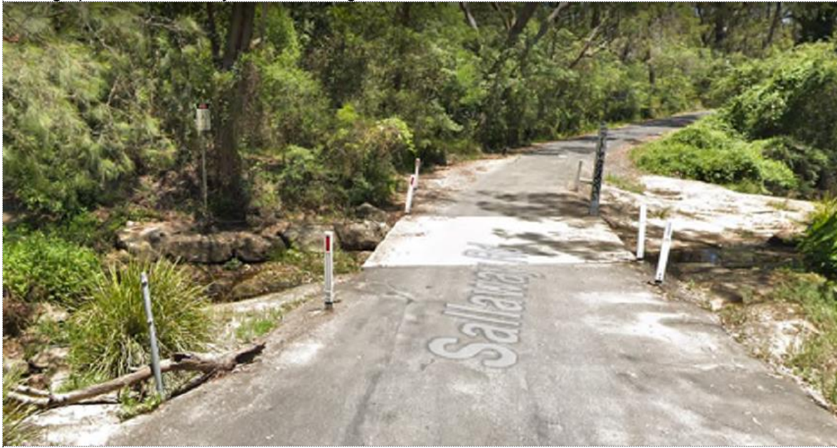
Street view of the culvert, January 2019 (Source: Google Street View).
