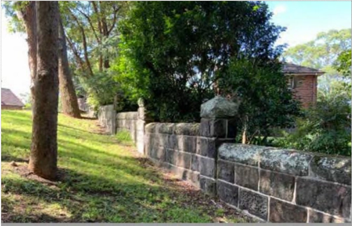
Sandstone block fence at 2 Beecroft Road
