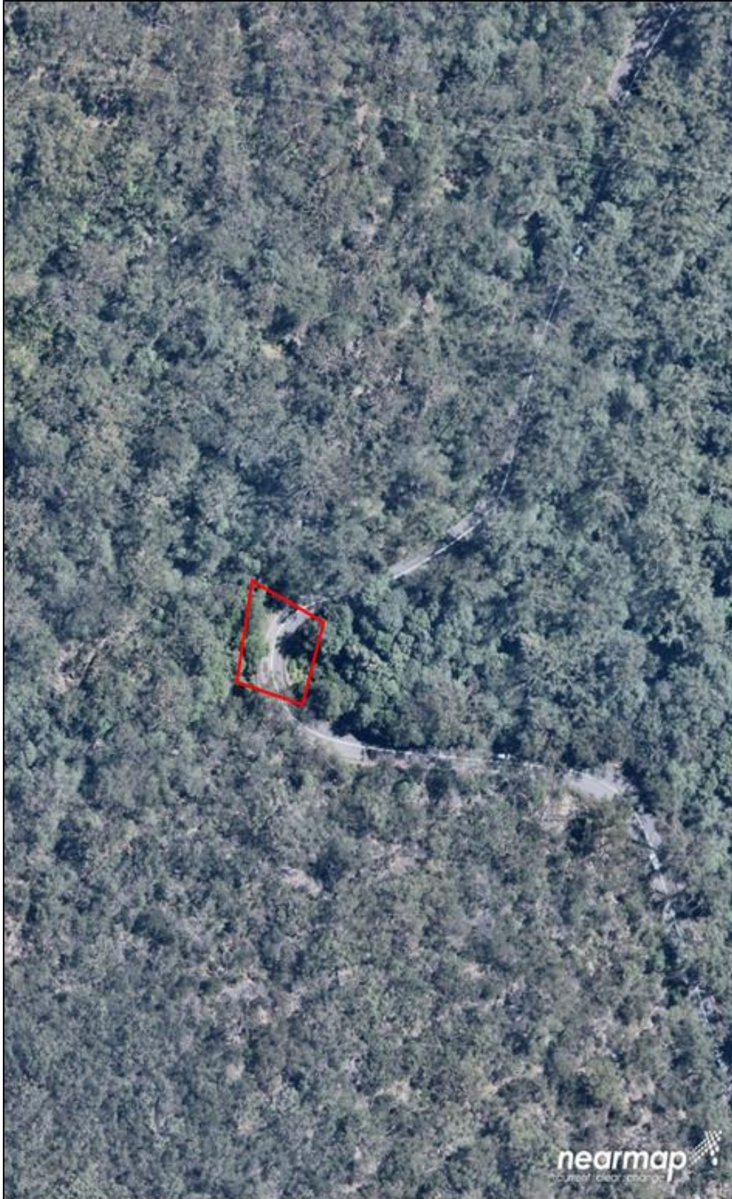
Aerial image of Galston Gorge culvert, Galston Road, Galston (source Nearmap).
