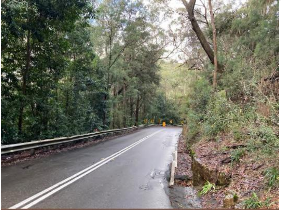
View of the culvert opening on the inner side of the road.
