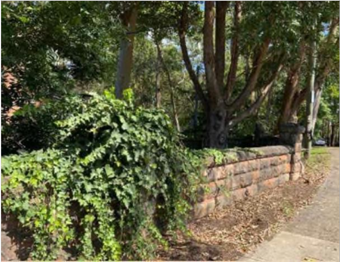
Sandstone block fence at 2A Beecroft Road.
