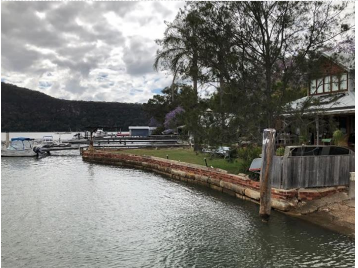
Photograph of the seawall, photograph taken 21.11.2017 (Source: Hornsby Shire Council).
