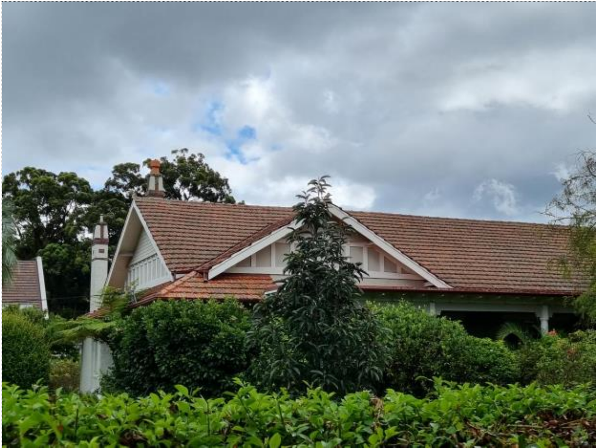
Side view of property
