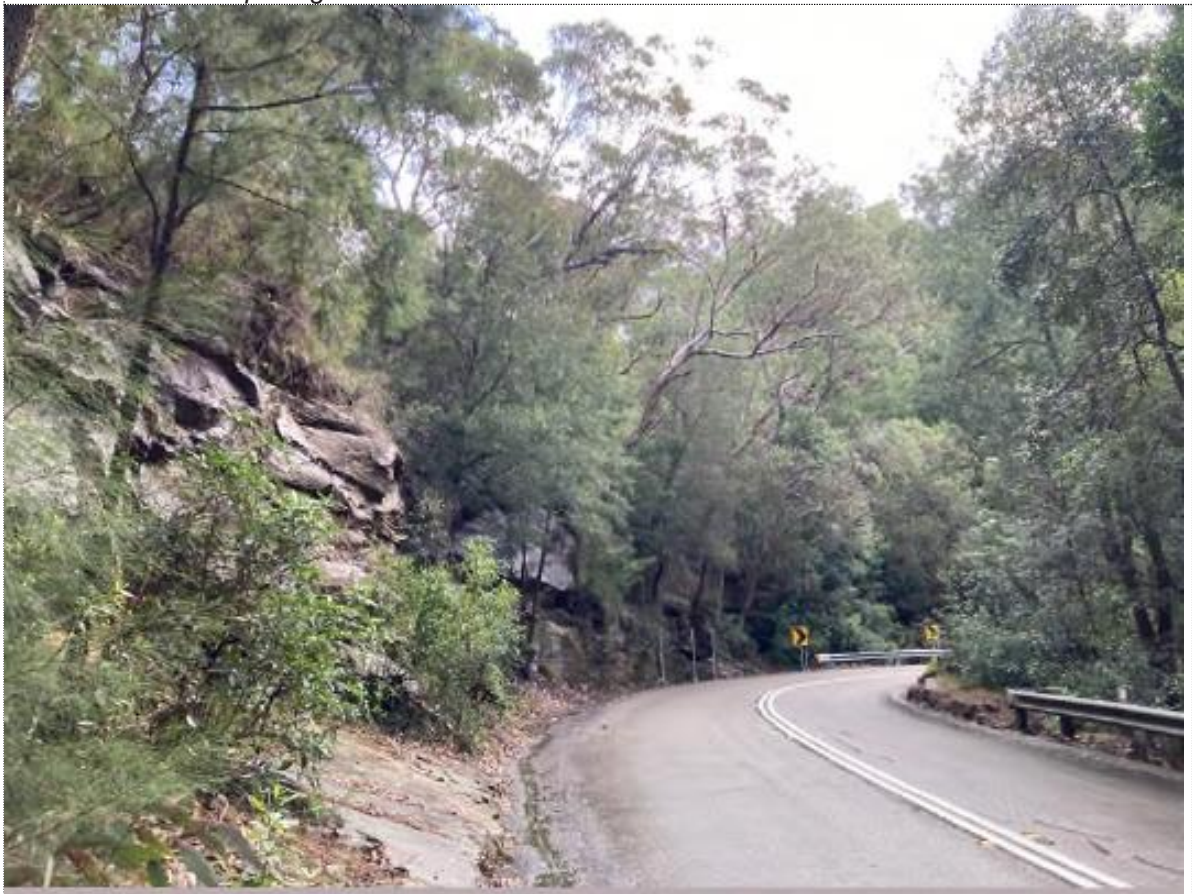
View west along Galston Road from the culvert.
