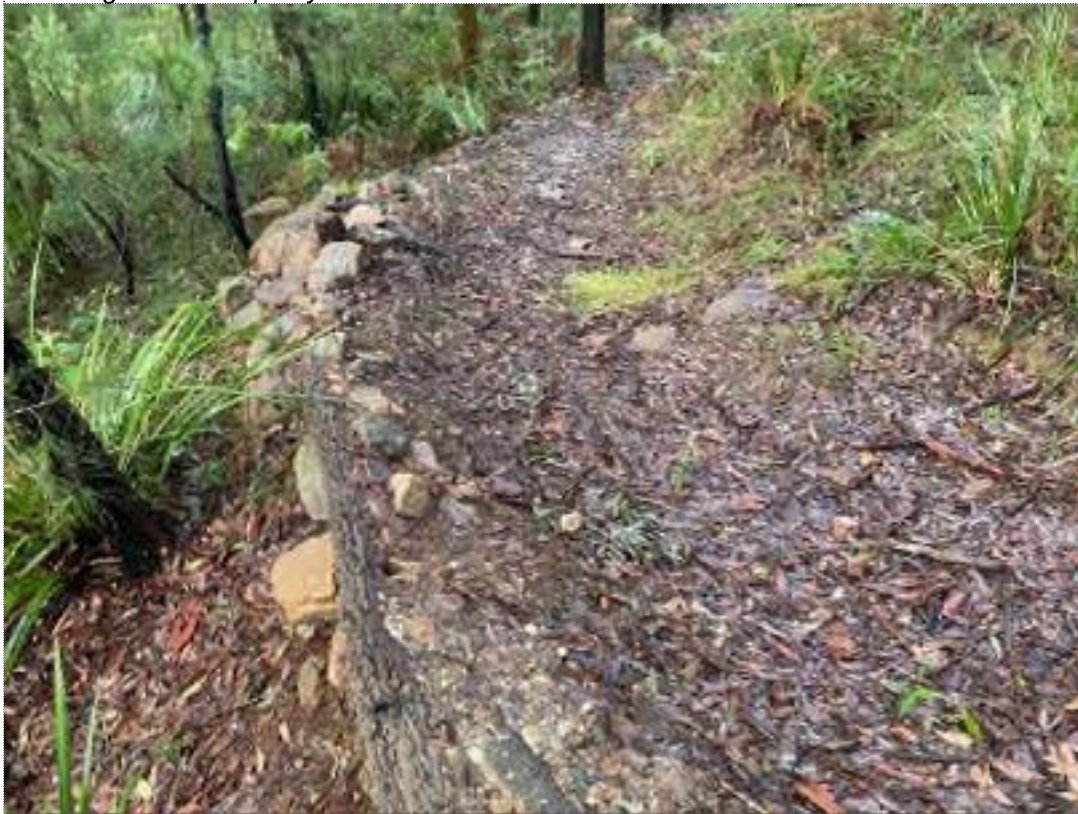
Terracing with sandstone and timber within the quarry.
