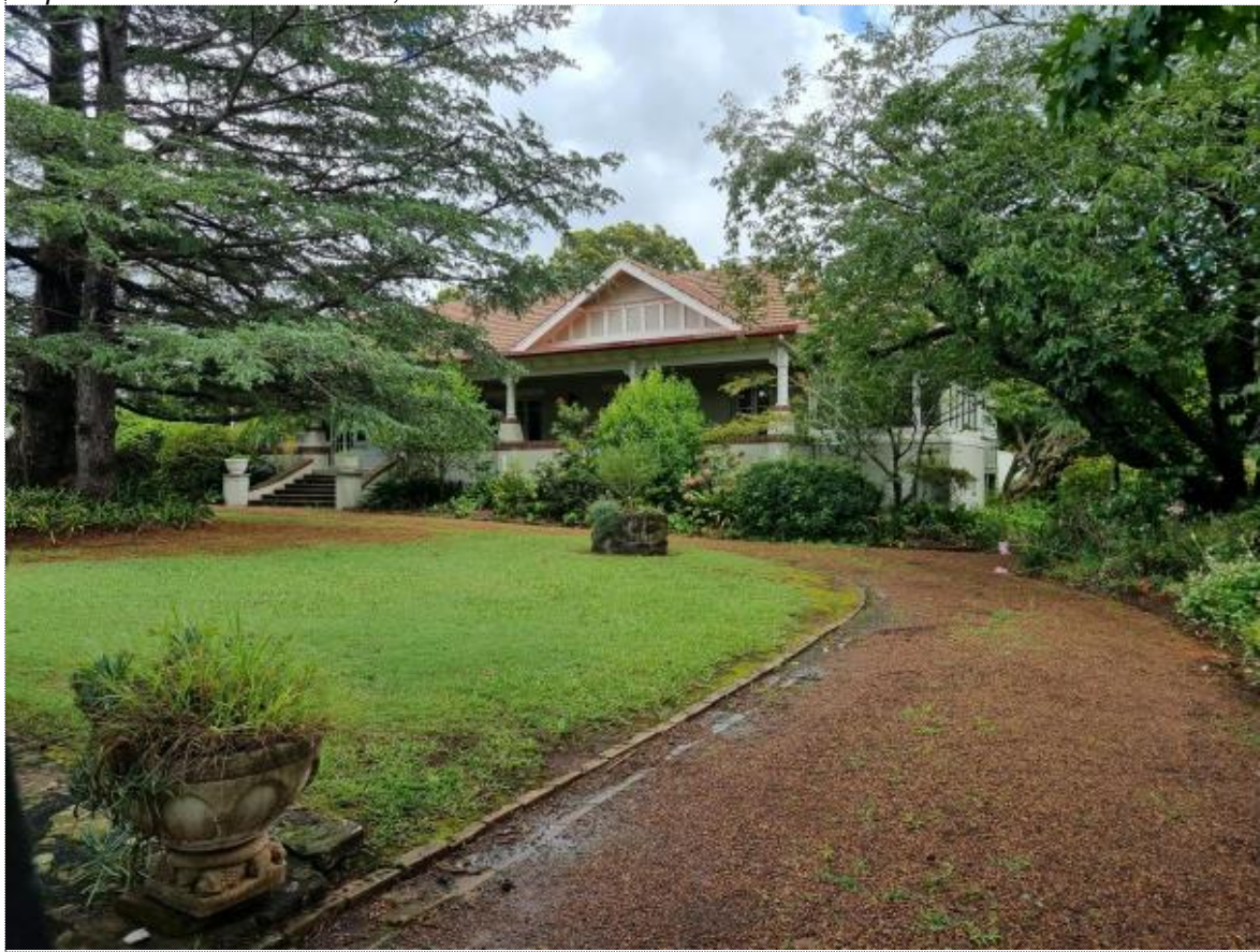
Front view of property
