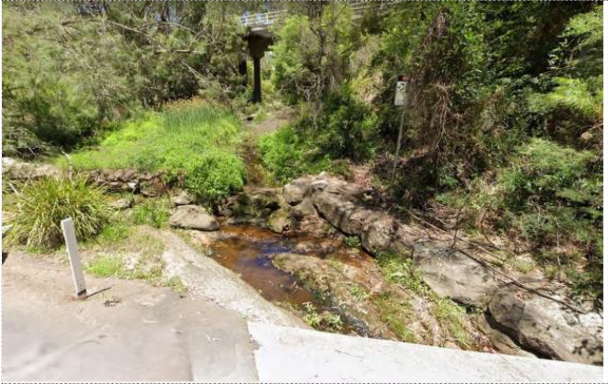
Photograph of the Sallaway Road crossing Colah Creek.
