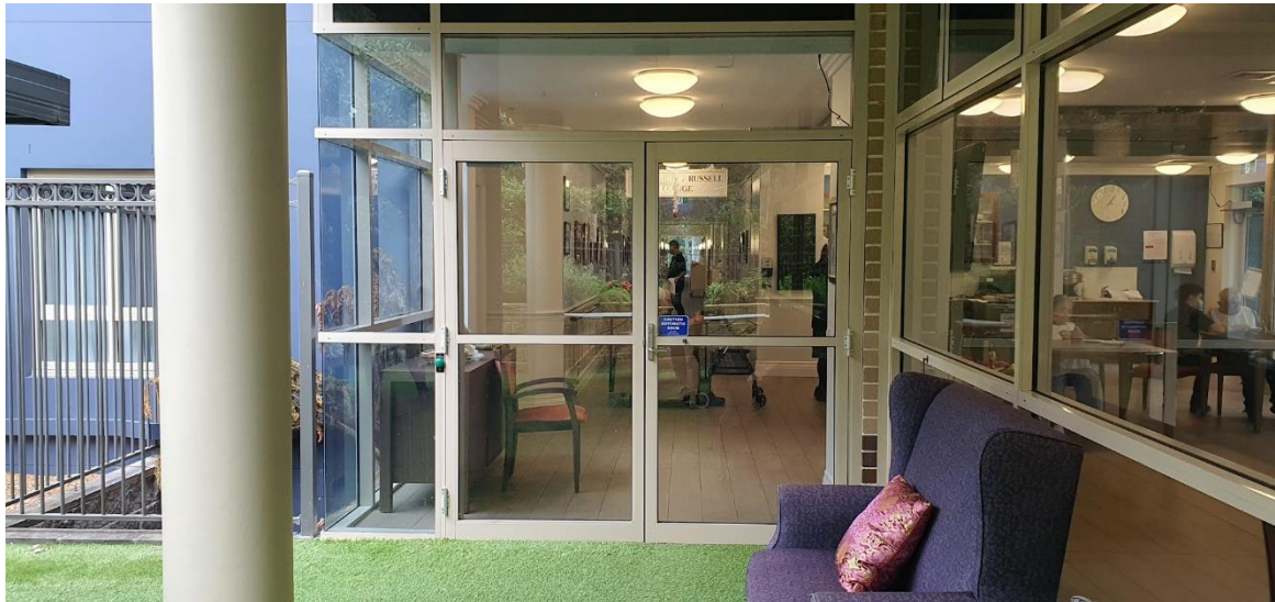
Photo 2: Door to be relocated
