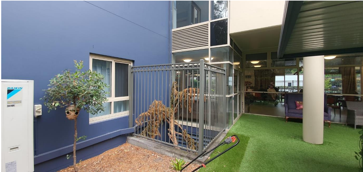
Photo 7: Window to be relocated
