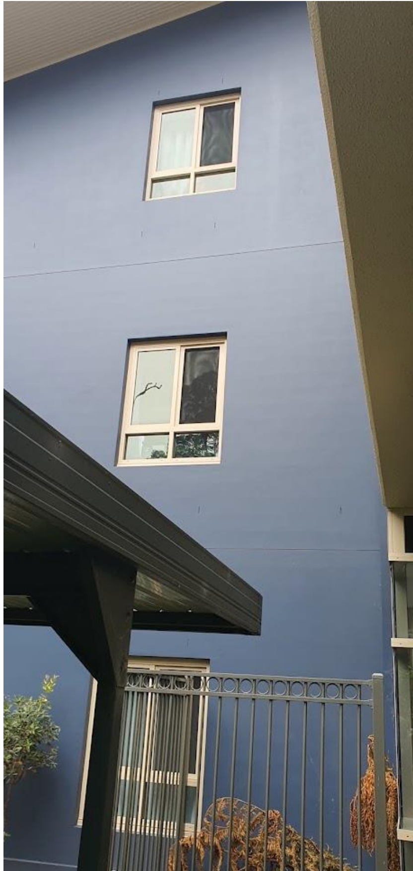
Photo 6: Lift to extend to top of existing building.
