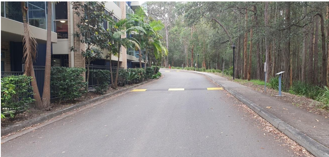
Photo 17: Building on left in relation to hazard on right.
